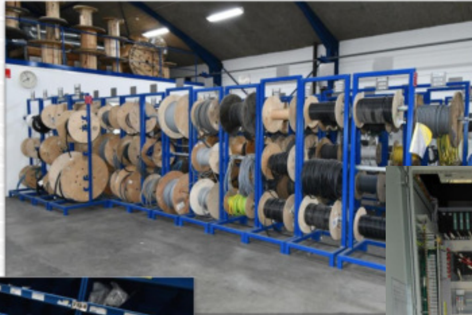
Control Cabinet Workshop
